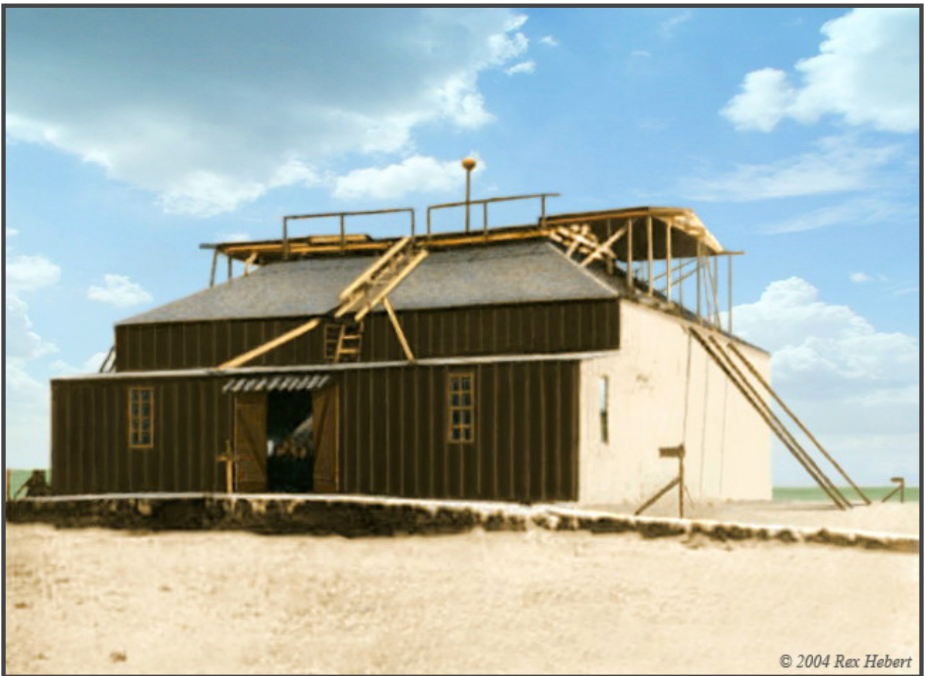
Tesla's Colorado Springs Experimental Station - early view "Experimental Station built to order by Joseph Dozier for World System Project" The barn-style building stood 50 x 60 feet with 18 foot ceiling From the center of the roof was a 200 foot pole fashioned with a 30" wooden ball covered in copper foil on top.
